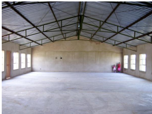
Interior of new building at Mpaka.
